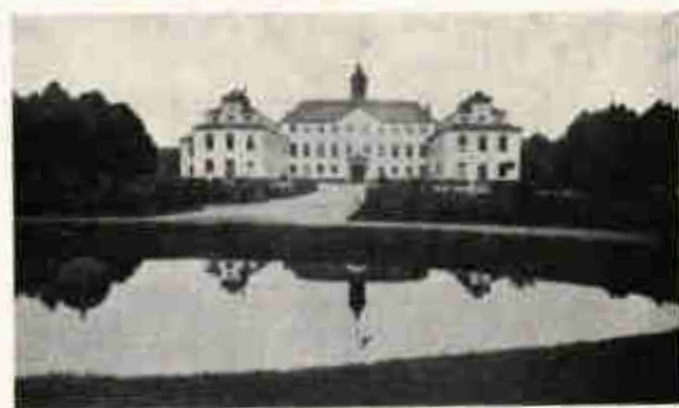
Fig. 11. Building on the main station.
