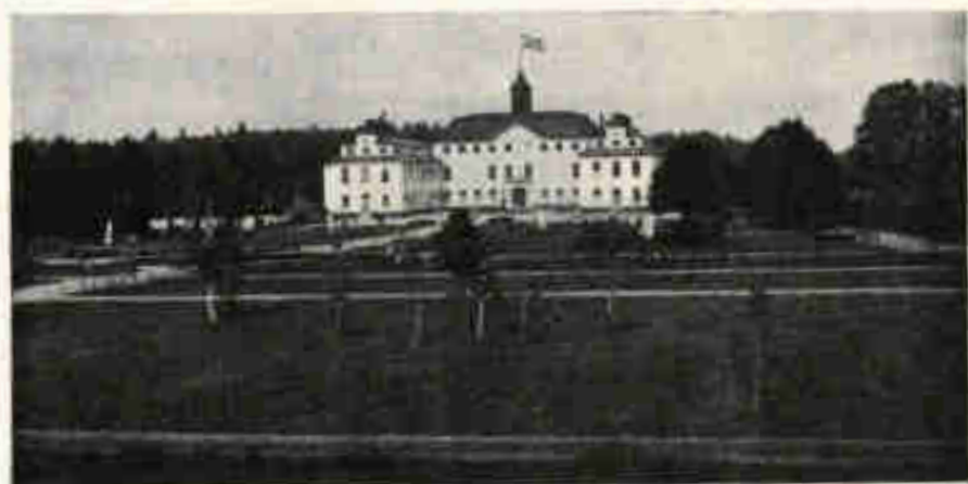
Fig. 10. Building on the main station.
